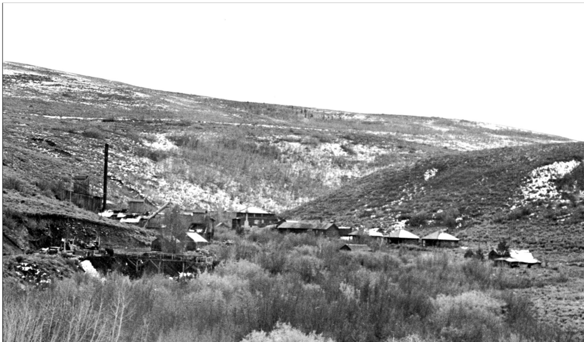
Figure 32. Paris Canyon Mine, about 1943, view southwest, showing portal and dump of Paris adit with mill and camp buildings of the McIlwee phosphate operation in the background. Photo from Wyodak, 1943.
