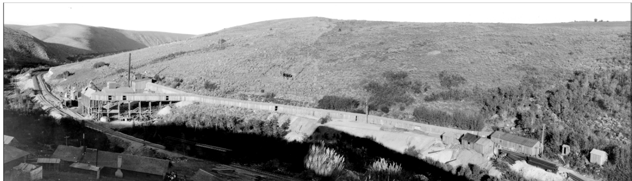
Figure 26. Overview of the Paris Canyon Mine showing the snowshed over the tramway, August 31, 1920. Photo by G. R. Mansfield, #478,479, USGS Photographic Library.
