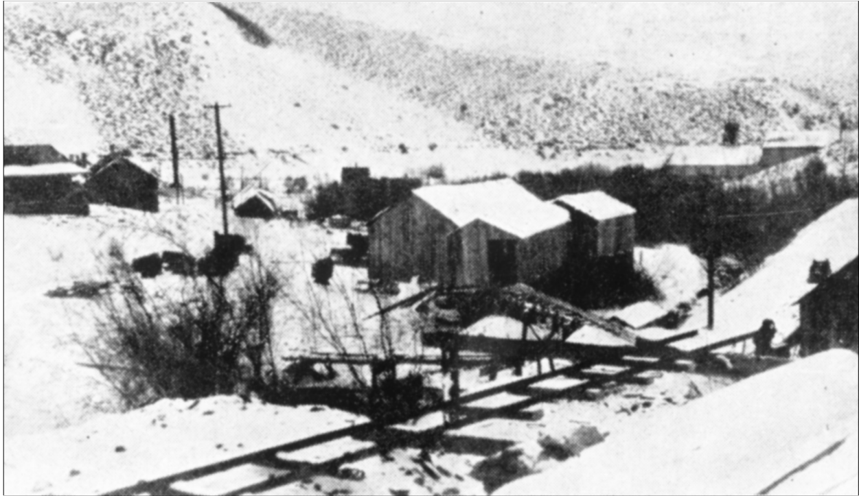
Figure 28. View from the Paris Canyon Mine entrance showing storehouse, employee's cottages, and part of the mill. This photo has been reprinted with the express written permission of Rock Products Magazine. Reprinted from the June 26, 1926 issue of Rock Products Magazine.
