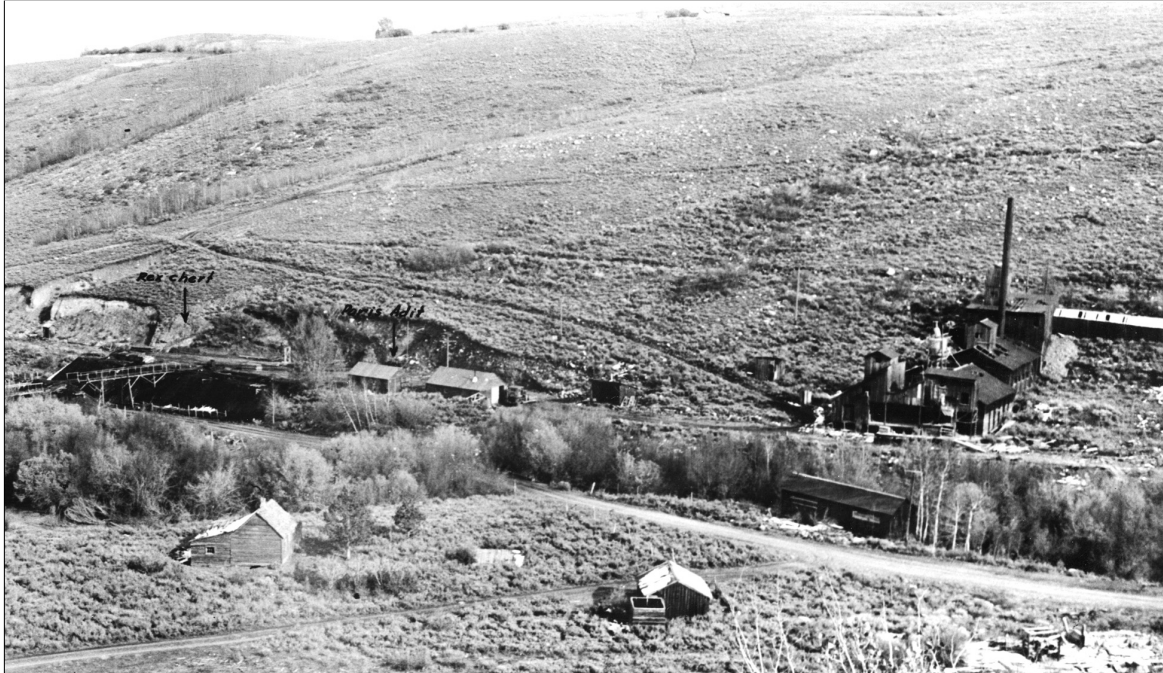
Figure 31. Paris Canyon Mine, about 1943, view southeast. The dump of the Paris adit and winze is at left. The mill of the old McIlwee phosphate operation is at right. Photo from Wyodak, 1943.
